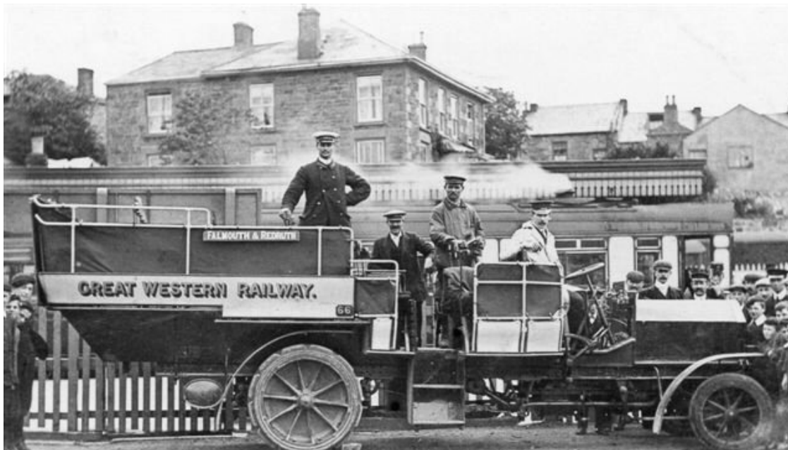
GWR Milnes Daimler 28hp open charabanc No. 66 (AF192) at Redruth Station. This type of body was known as a Lee seater charabanc with several points of side access and stepped floor and removable canvas upper sides, primarily for touring / sightseeing. [© Chris Heaps Collection]
